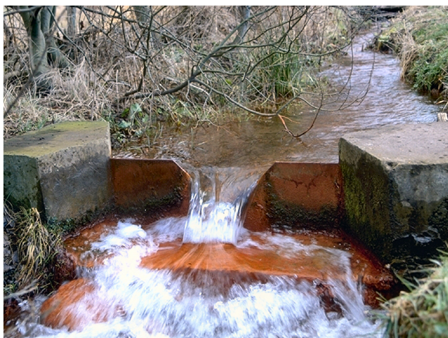
Figure 15. Example of a V-notch weir measuring the overflow from the Blaydon Hazard Shaft, an abandoned coal mine near Newcastle upon Tyne, UK
